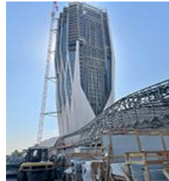
Figure 3: Central Bank of Iraq (CBI) building in Al-Jadriyha- the source is the Researcher
