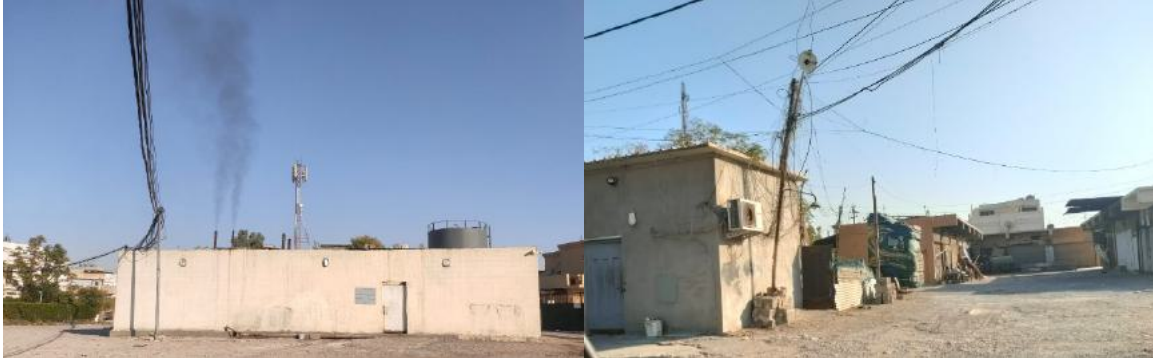
Figure 13. Neighborhood diesel generator on a mid-road pavement and redundant utility support insulators in the Kuran neighborhood of Erbil City.
