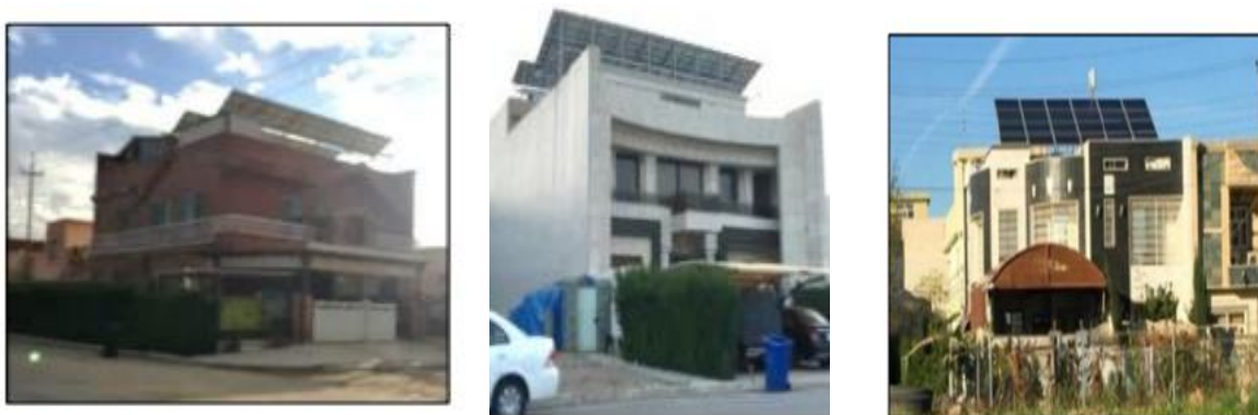
Figure 9. Houses in Erbil city with installed PV system
