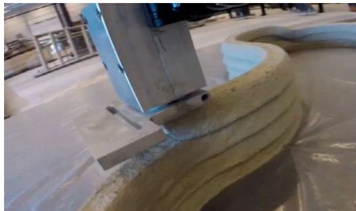
Figure 2. The construction process uses Concrete Printing technology (Bos et al., 2016)
